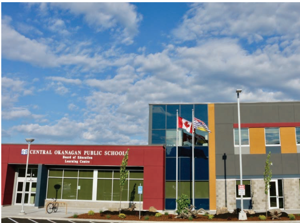
New Modern Facility for Central Okanagan Administration. Many years of planning came to fruition when the new Central Okanagan Public Schools Board of Education Learning Centre was opened in March 2018. The new administrative office is located at: 1040 Hollywood Road South. The Central Okanagan Public Schools Board of Education Learning Centre is open from 8am to 4:30pm, Monday to Friday. The telephone number remains the same.(250.860.8888)
